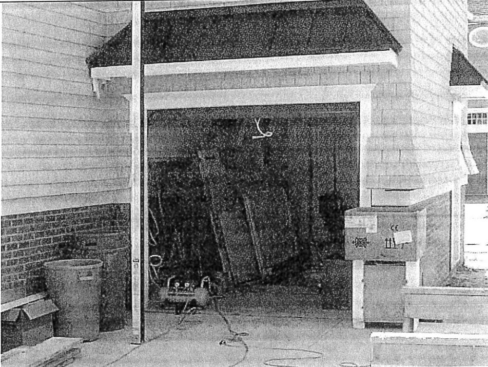
View: Garage Area (Note: Open Wall to Crawlspace/Storage Area on the left)
